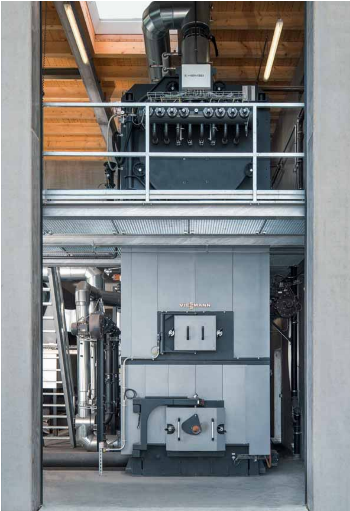
Holzwerk Schilling Rot an der Rot, Germany Vitoflex 300-SRT, 1700 kW Woodworking industry
