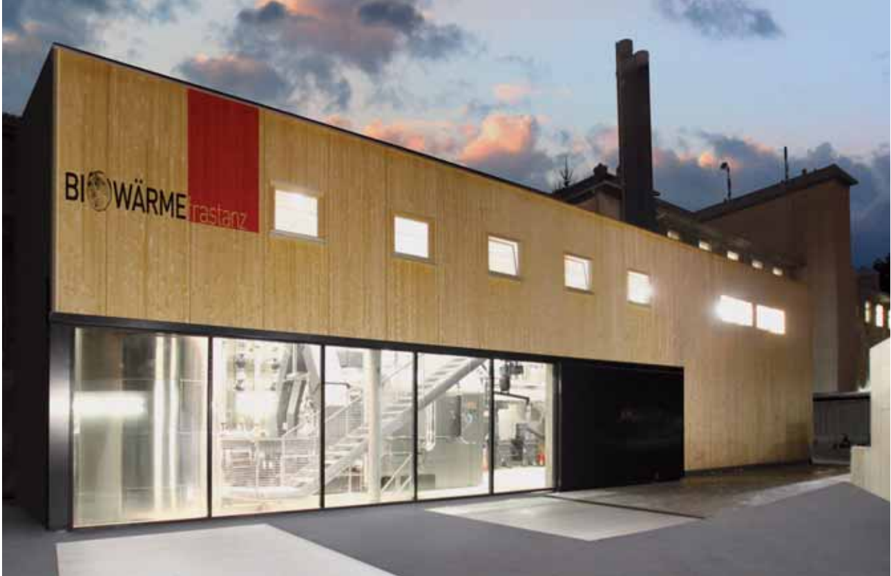
Bioheating centre at E-Werke Frastanz, Austria
