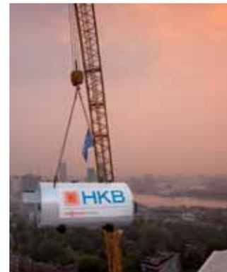
Installing a boiler through the roof of a 120 m high building
