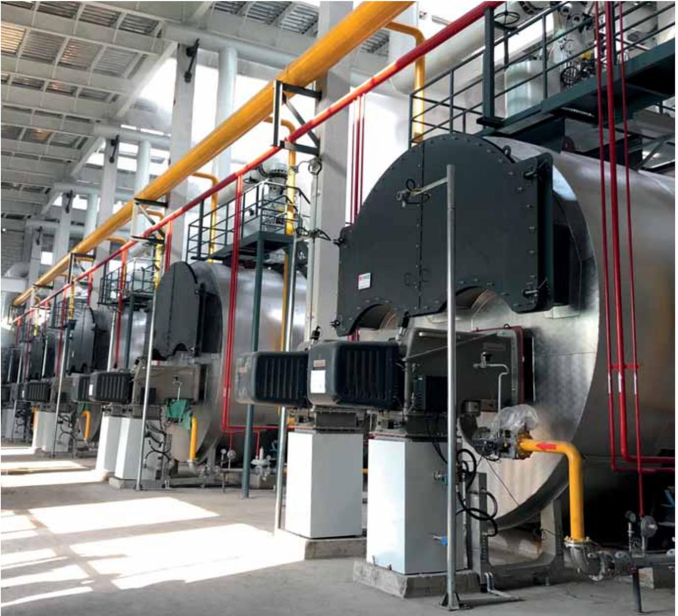
Five Double flame tube boiler Vitomax D
